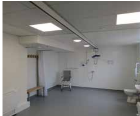
Two spacious changing rooms with overhead tracking hoists directly to the pool side and shower areas.
