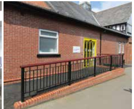
A new ramped entrance for easy wheelchair access.
